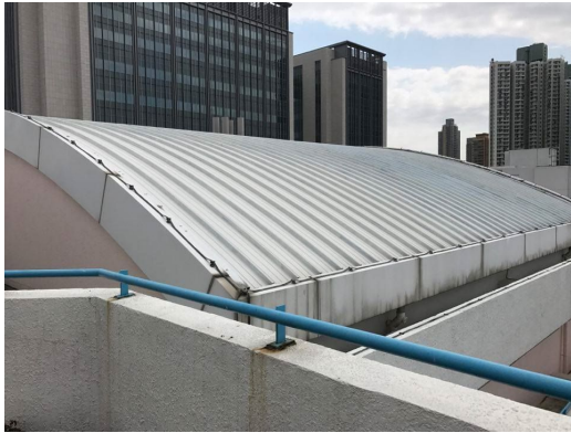
Thermal Insulation Coating on the rooftop of the school library
